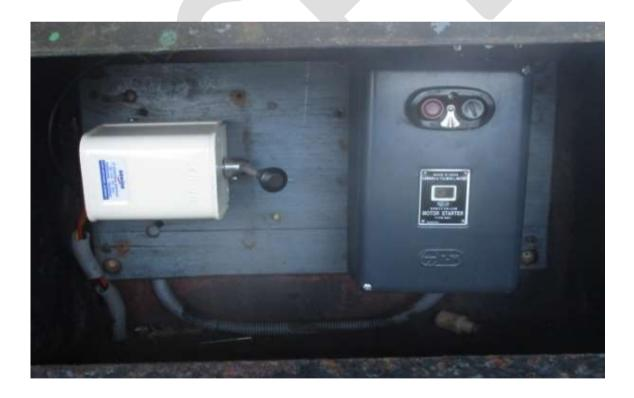
Fig 2.5 Reverse/Forward switch and starter/stopper
