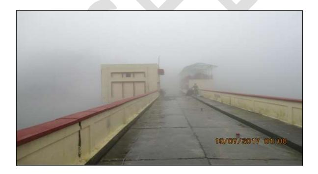
Fig 6.2 Dam top road after providing wearing coat
