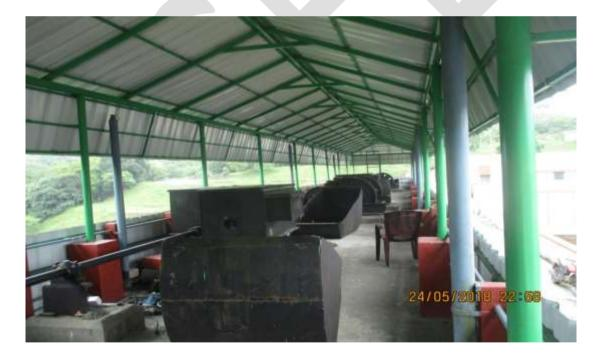
Fig 6.4 G I sheet roofing for spillway gate controlling platform
