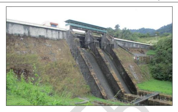
Fig 6.3 G I sheet roofing for spillway gate controlling platform
