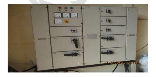
Fig 2.18 Main panel Board in Intake
