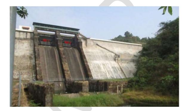
Fig 2.16 Spillway of Kuttiadi Dam
