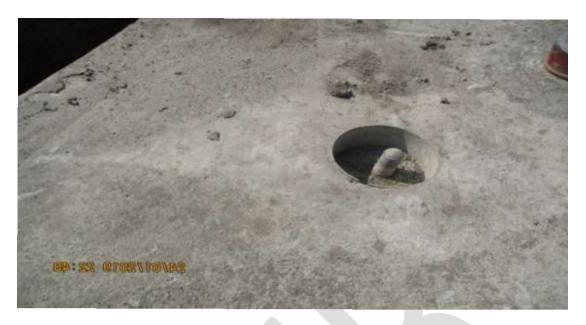
Fig 5.1 Location of station for Deformation measurement
