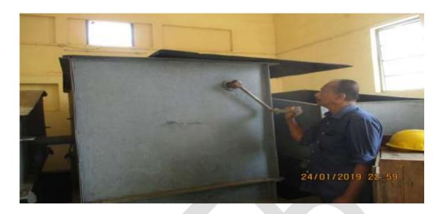
Fig 2.19 Manual operation of gate
