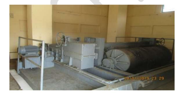
Fig 2.9 Scour gate hoisting system
